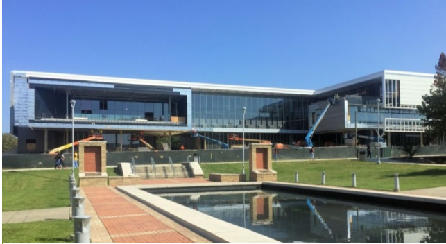
New student center under construction.
