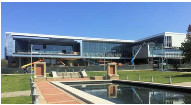
New student center under construction.
