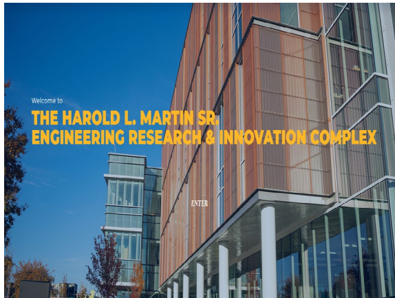
Harold L. Martin Sr. Engineering Research and Innovation Complex, completed in fiscal year 2022.
