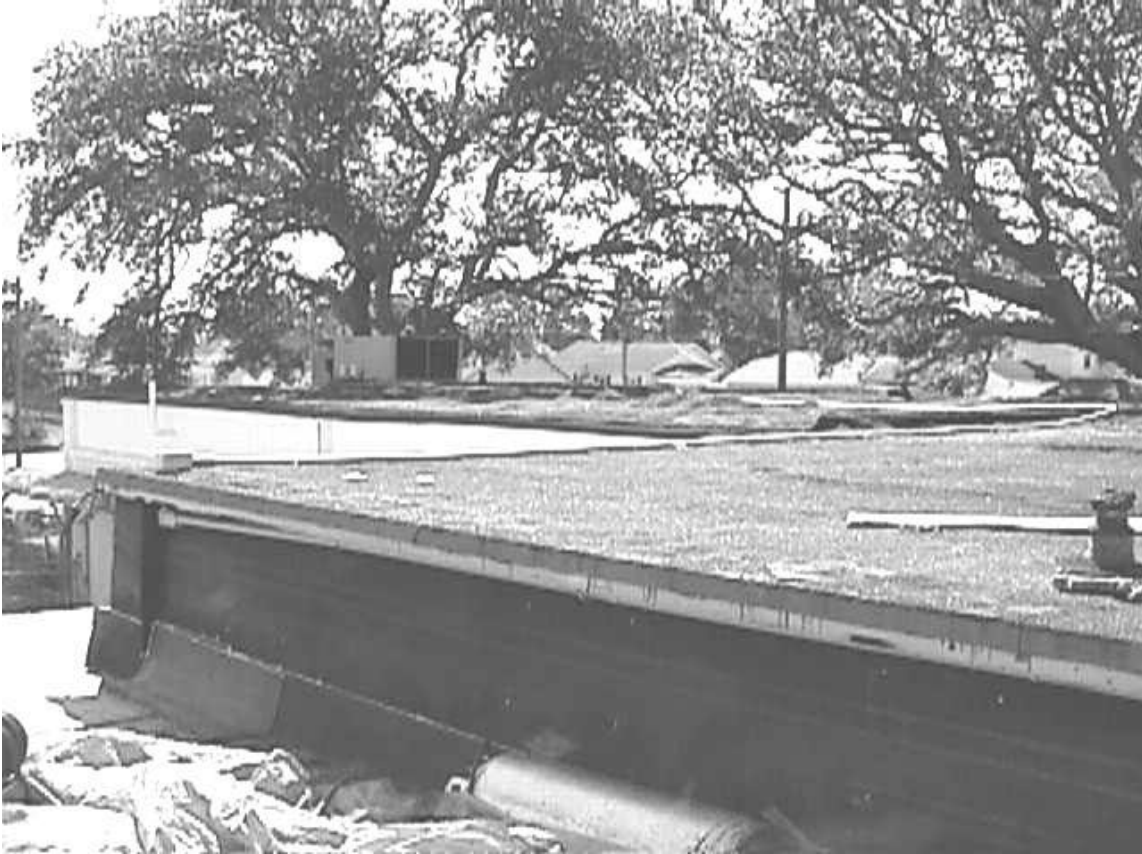
Beaufort Head Start Center Roof
