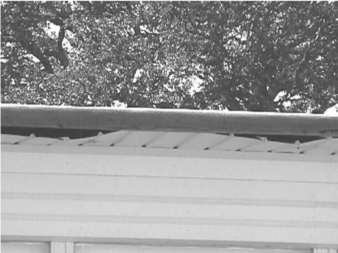
Beaufort Head Start Center Roof
