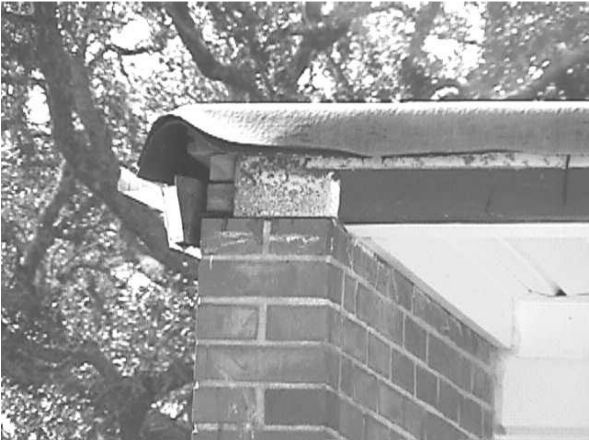
Beaufort Head Start Center Roof
