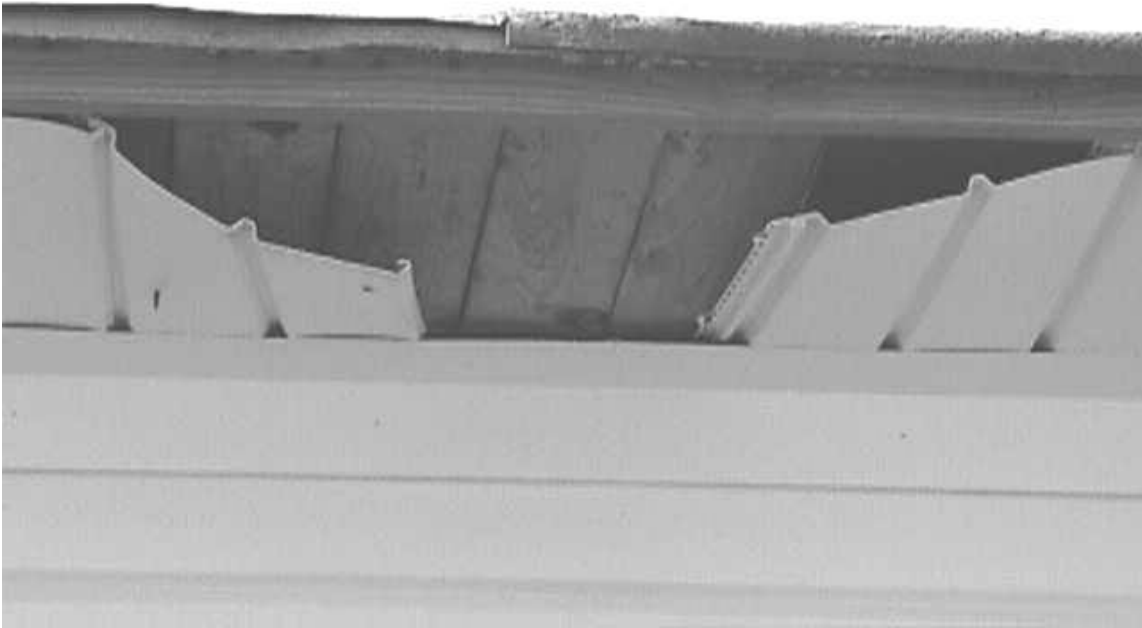
Beaufort Head Start Center Roof
