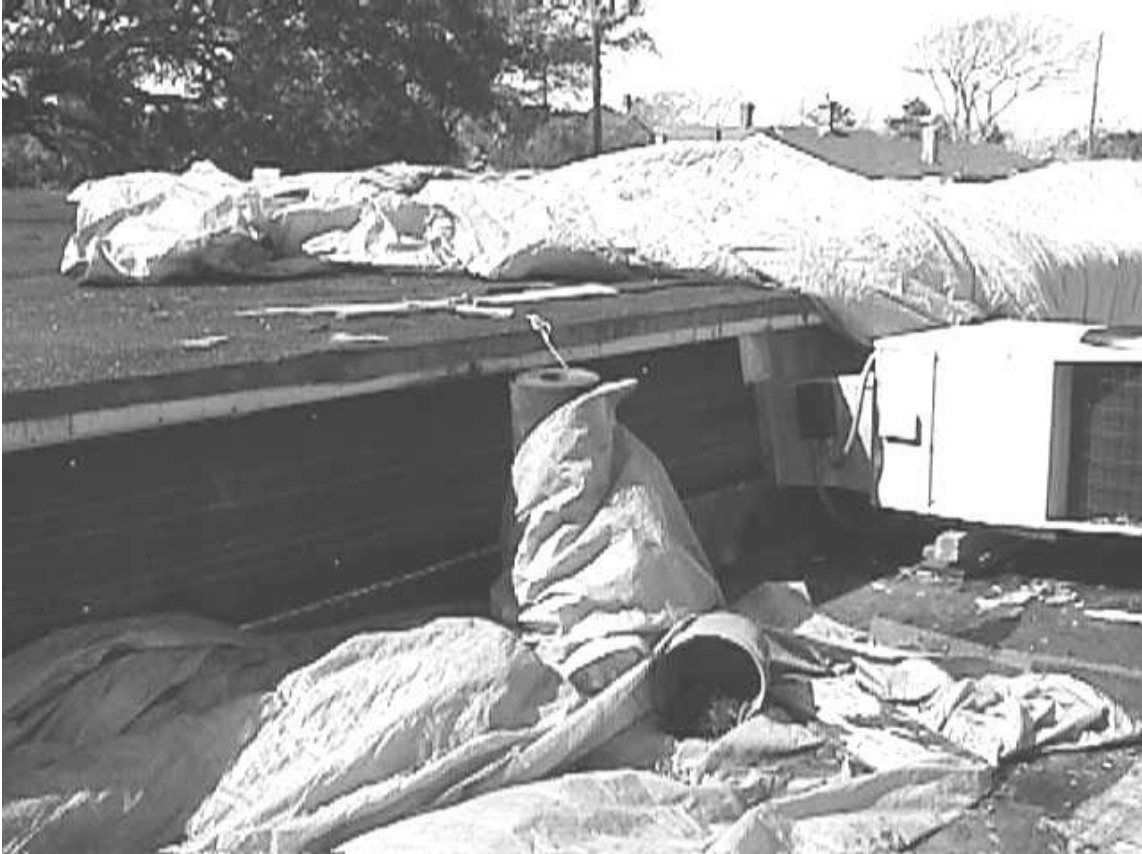
Beaufort Head Start Center Roof
