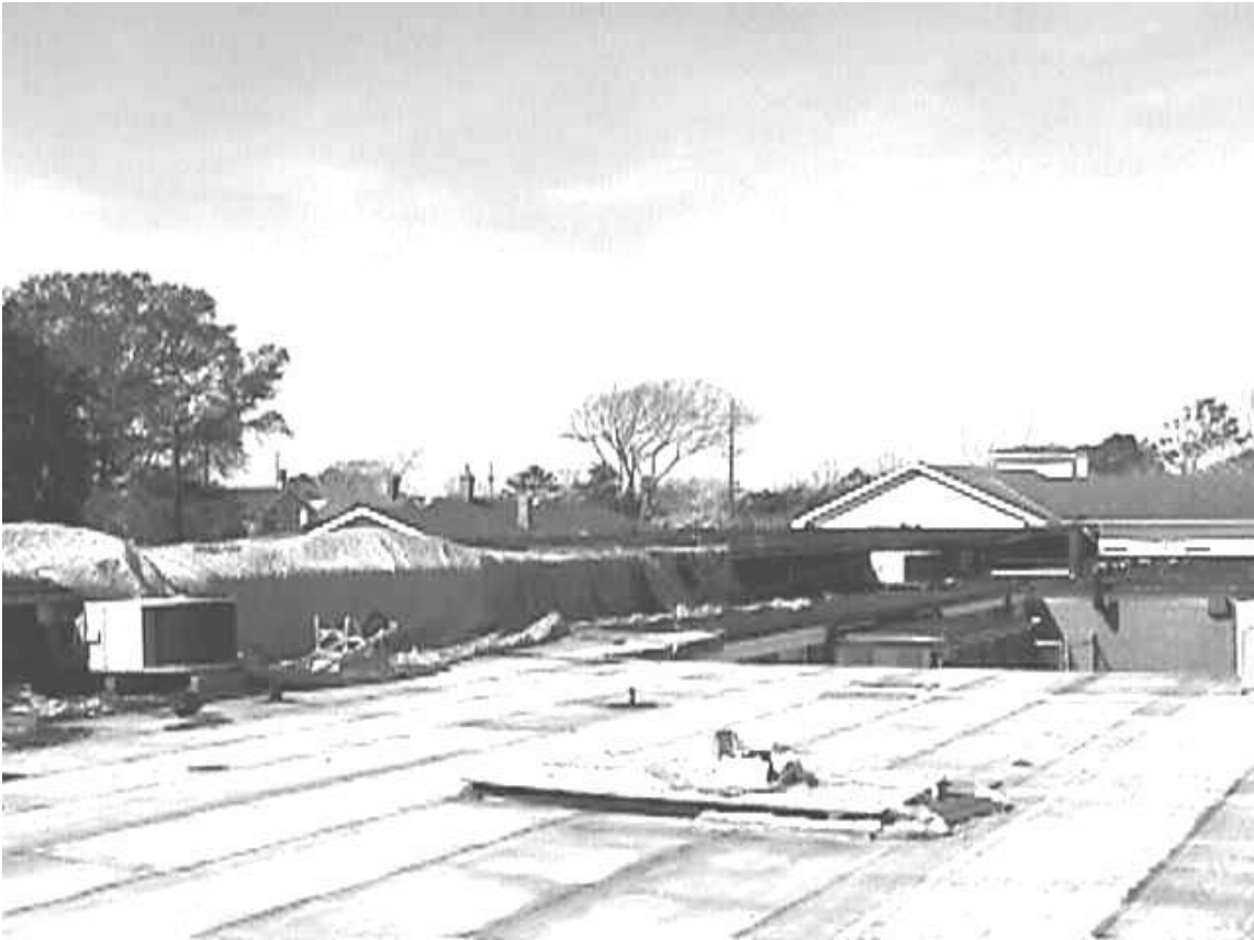
Beaufort Head Start Center Roof
