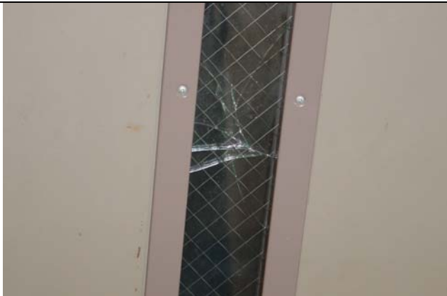
Cottage Dorm Door Damage
