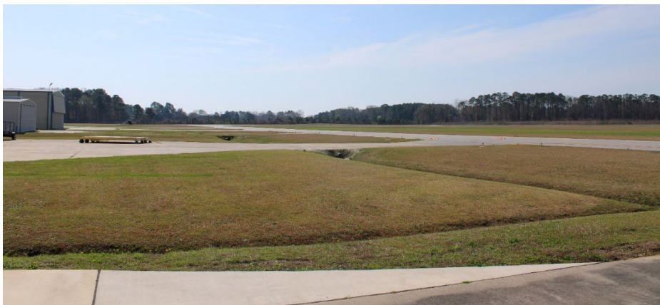
Figure 5: Taxiways to access hangar build sites (1,200 feet by 100 feet), March 11, 2026. Photo by OSA.
