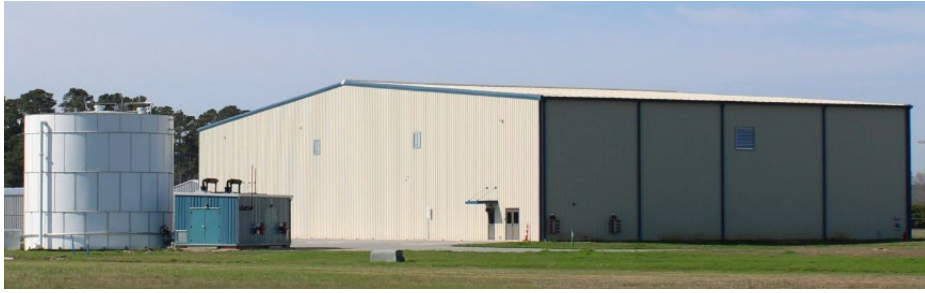
Figure 3: Corporate jet hangar with associated water tank and fire suppression system, March 11, 2026. Photo by OSA.
