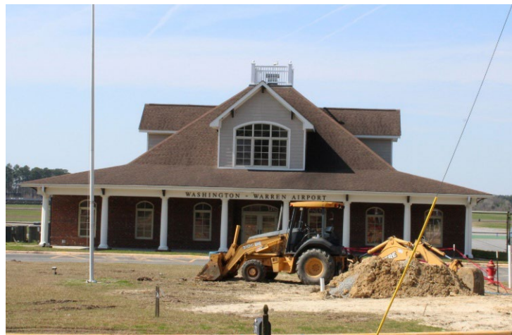
Figure 1: Washington-Warren Airport terminal building, March 11, 2026. Photo by OSA.
